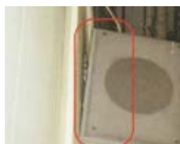
拡声装置の取付不良❖ 3
